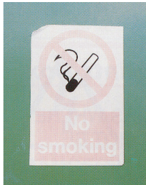
Safety sign is fading and peeling.
